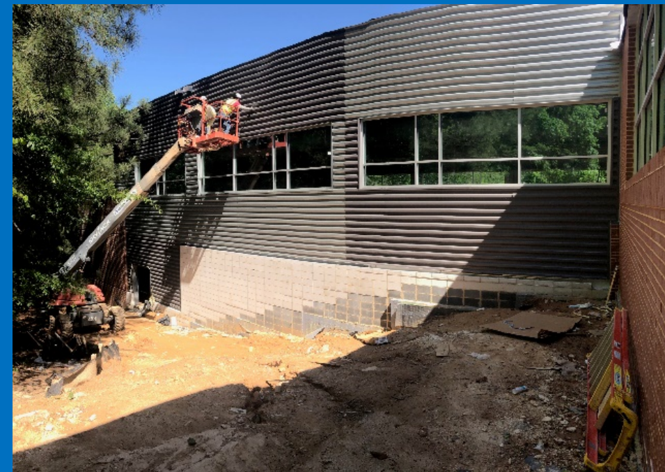
West Elevation Metal Panel Installation
