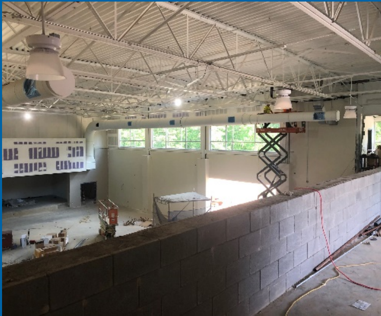
Gymnasium Light Fixture Installation
